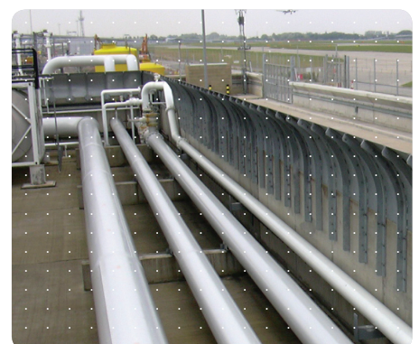
Below: Wave deflecting bund wall
