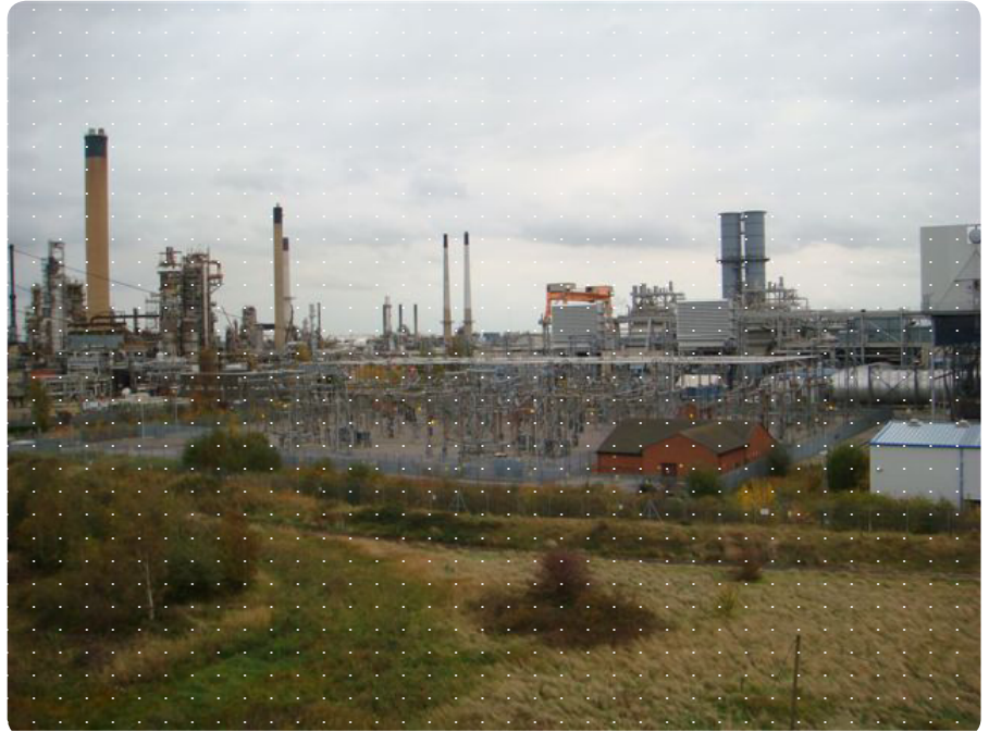
The Power Station in Essex.
